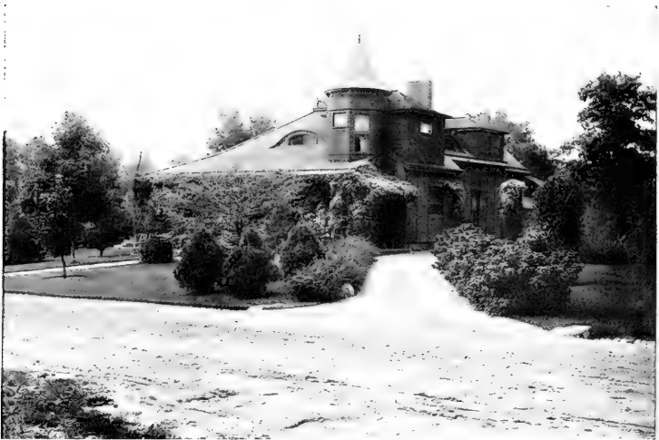
The house in 1900, showing improvement in front lawn by the massing of shrubbery
